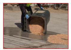
The rest of the sawdust or sand can be placed over the oil or chemical spill to help contain and absorb it.
