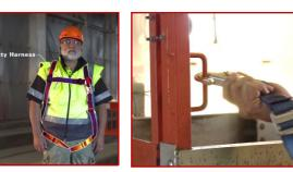
A safety harness needs to be worn not only in Boom Lifts, but also Scissor Lifts that have certified anchor points installed.
