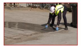
The drain covers should be placed over the affected drain and a dam of sawdust or sand applied.
